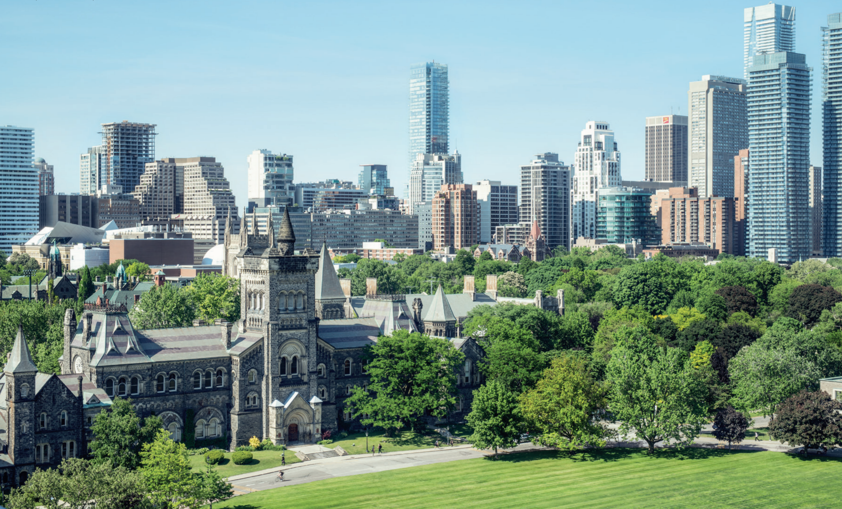
A view of University College and Bloor St. and Yonge St. from the Dr. Woo Hon Fai Terrace on Level 8 of the Myhal Centre. (Photo: Daniel Ehrenworth)
