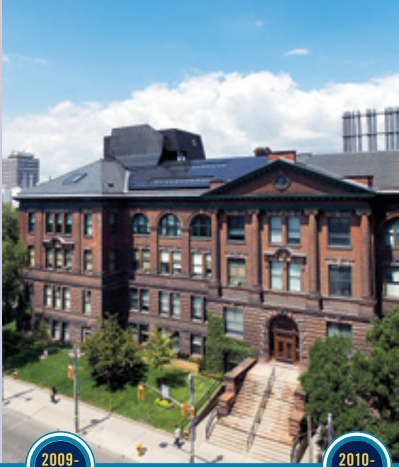
The Lassonde Mining Building with an exterior view of the transformed fifth-floor addition.
